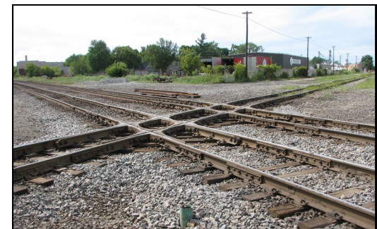
North and South, East and West Rails cross, creating the Diamond of the "Diamond District".
